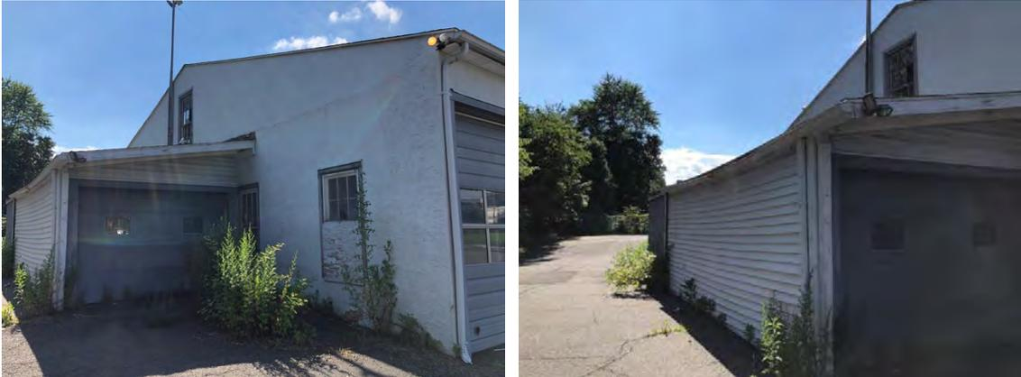
*Figure 8: Sagging rooflines.*
