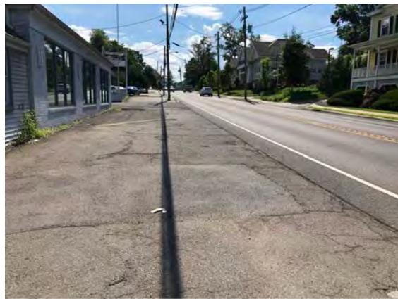
Figure 25: Cracked pavement.
