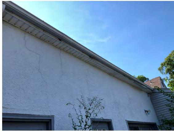
*Figure 13: Cracks in stucco suggest developing structural issue.*
