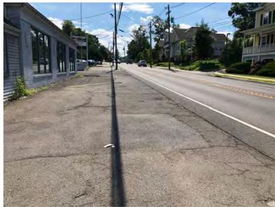
*Figure 25: Cracked pavement.*
