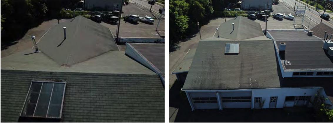
*Figure 11: Aerial imagery suggests roof leakage.*
