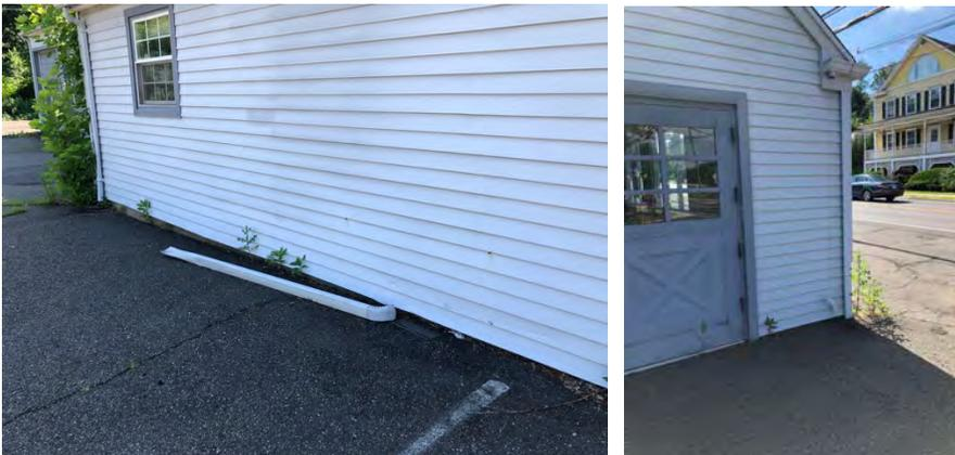
*Figure 9: Damaged gutters and/or downspouts.*
